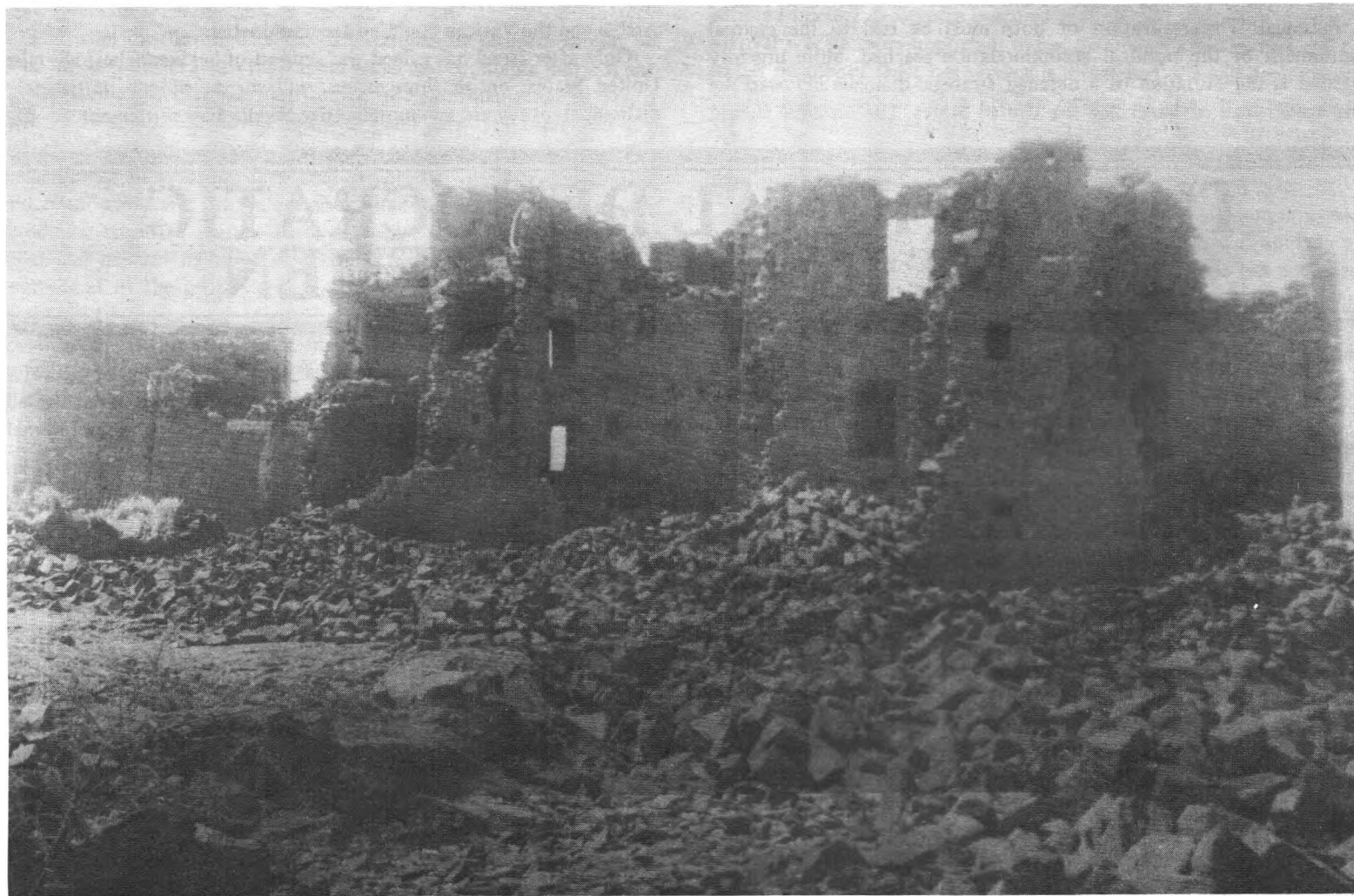
North Yemeni village completely destroyed by the regime's forces
