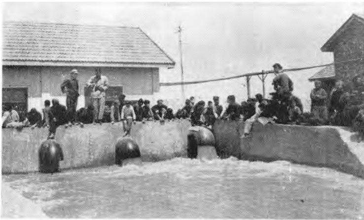
Local efforts complement big conservancy projects. This pumping station in Tanyang County, Kiangsu, irrigates 8,500 hectares
