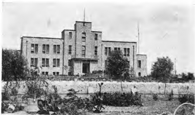
The three-storey main office was constructed with bricks made on the farm
