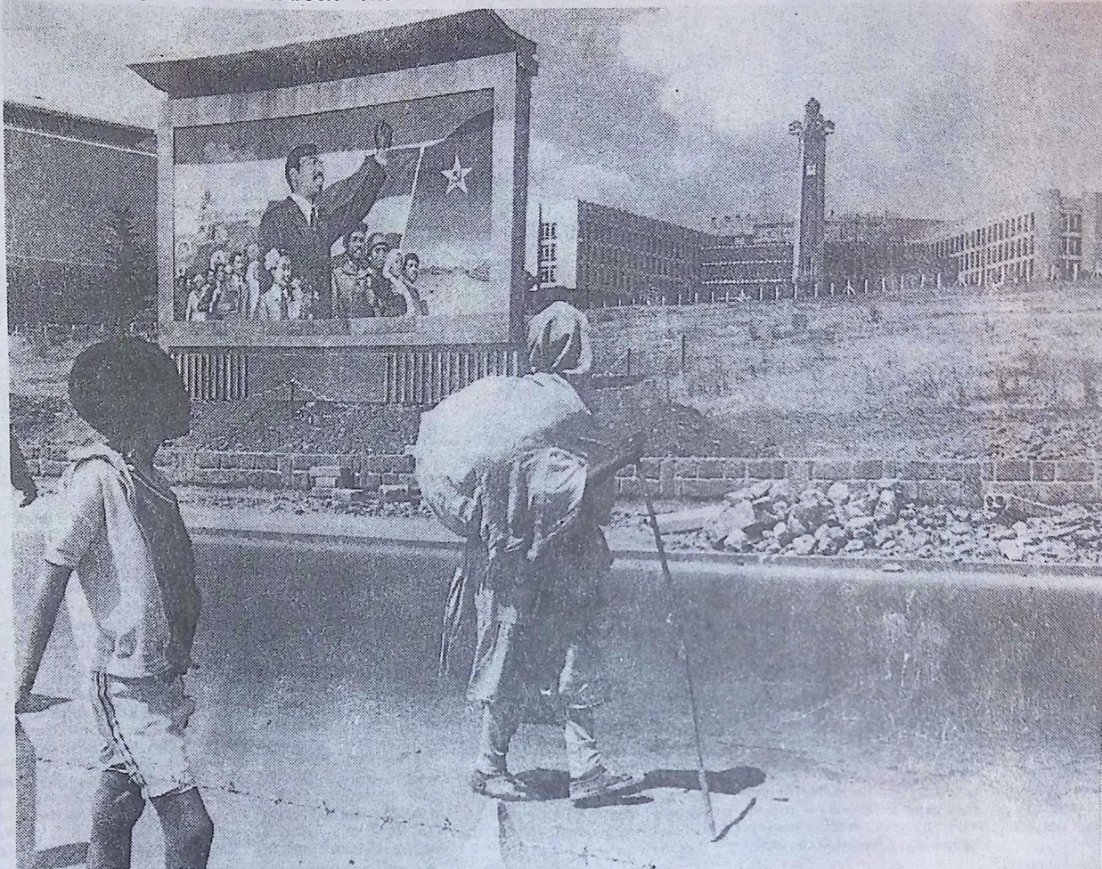
Municipal Buildings in Addis Ababa, a hoarding commemorates the 1974 revolution
