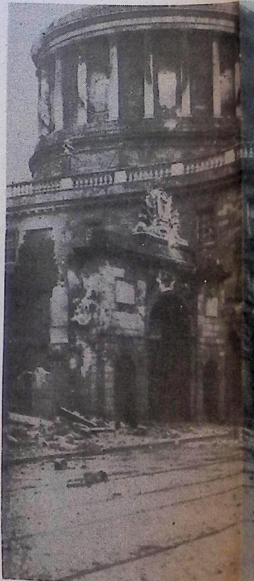
Battle damaged Four Courts in Dublin
